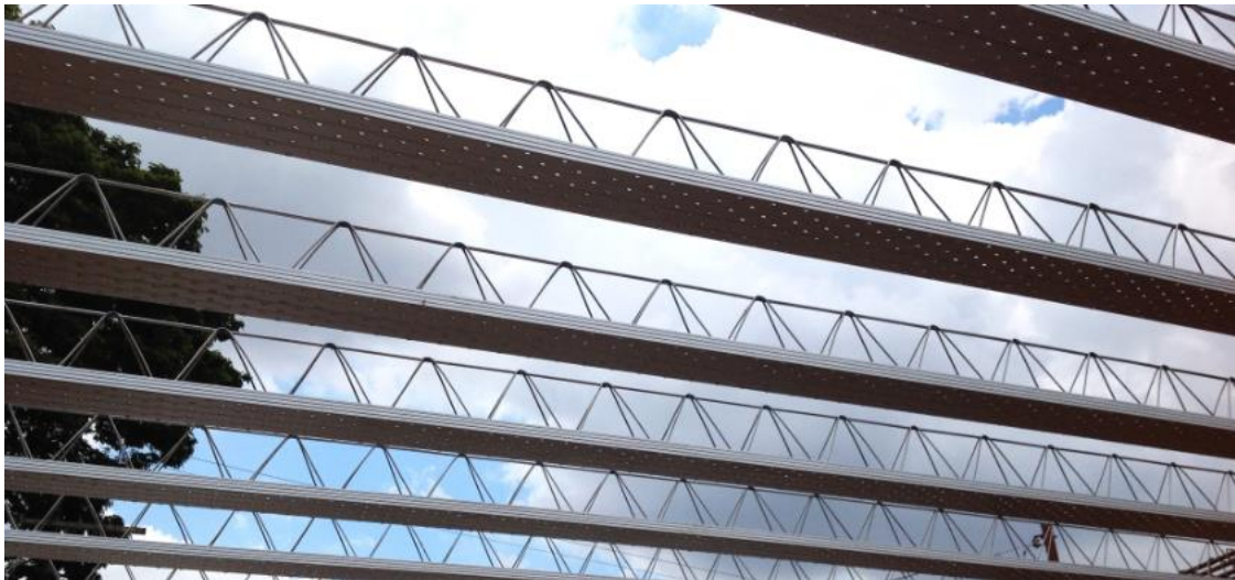
Figure 1.5 — Composite ribbed slabs featuring the Trelifácil® solution.
