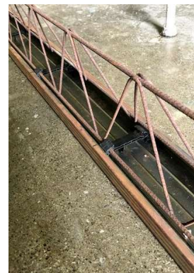
Figure A.2. Preparation of CFS shuttering, evidencing the connection to rebar truss. Source: Author.
