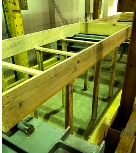
Figure A.1. Preparation of wood formworks before concrete casting. Source: Author.
