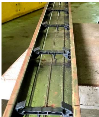
Figure A.2. Preparation of CFS shuttering, evidencing the connection to rebar truss. Source: Author.
