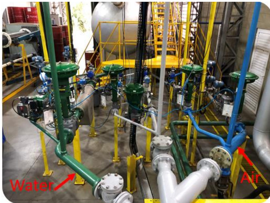
Figure 20 - Single-phase measurement split-range configuration photography (Source: author)
