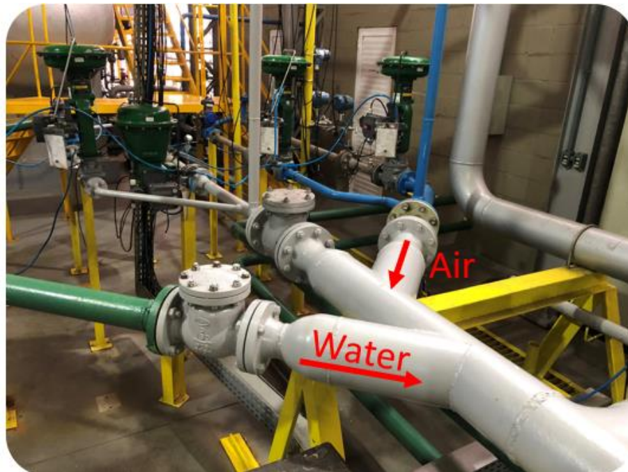
Figure 23 - Original mixing arrangement (Source: author)
