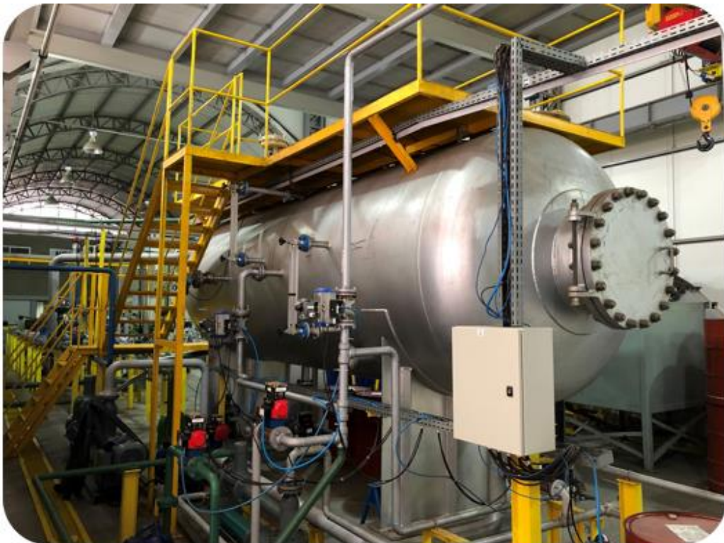
Figure 17 - Separator vessel photography (Source: author)
