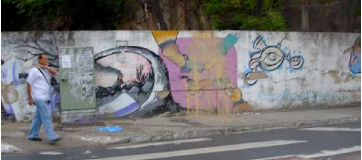
Fig. 103 – Muro com graffiti [E.20]
