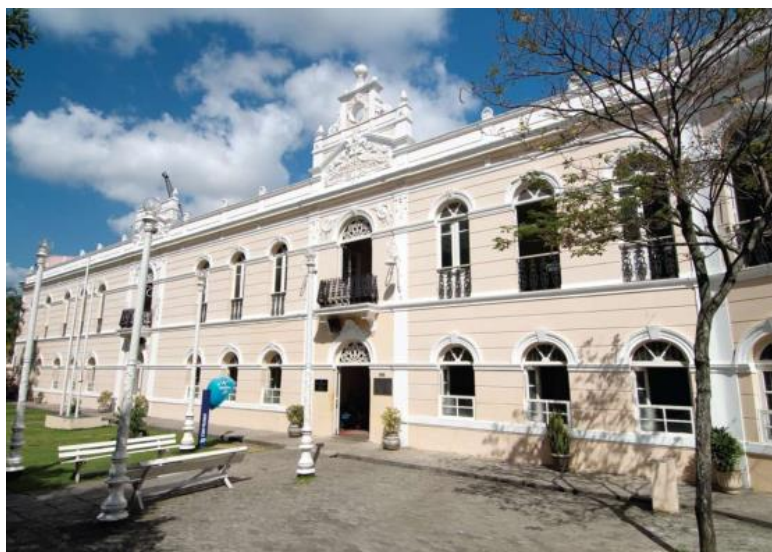
Figura 16 – Fachada Principal (Leste) da “EEEFM Maria Ortiz”
